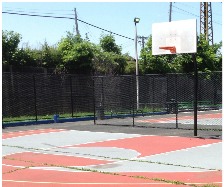
Figure A3: NYCHA South Jamaica Houses cloudburst pilot. The existing basketball court will be excavated to create underground water storage and repair the surface. The new “cloudburst” design will lower the basketball court, allowing it to fill with water during extreme rain, and providing a new seating area for residents
