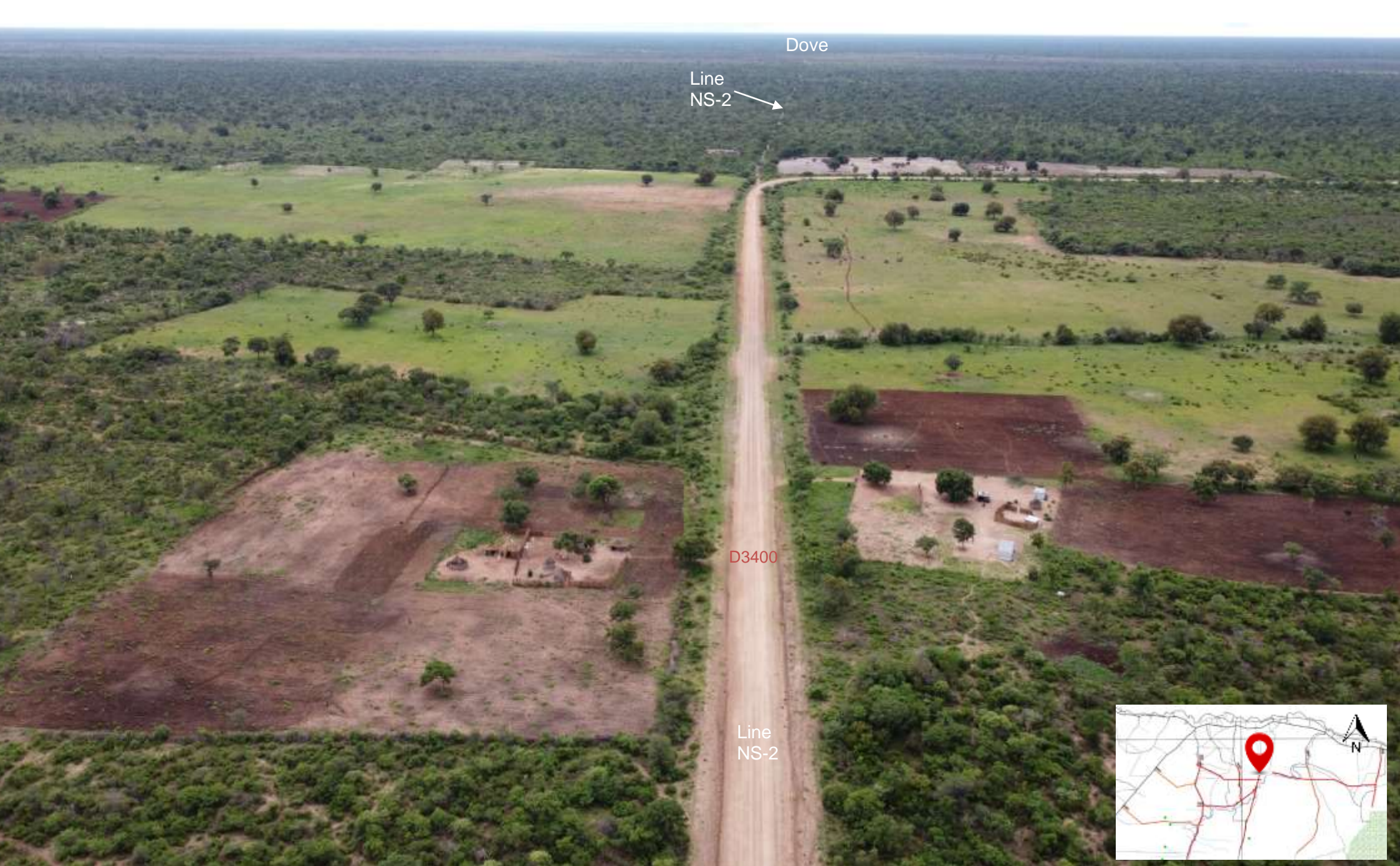
Plate 1.7: Middle section of the proposed 2D seismic survey Line NS-2 detailed location shown by a drone aerial view to the north along the D3400 Road towards junction with the existing tracks linking Dove to the D3400.
